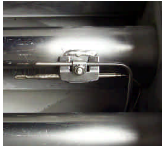
Typical high-limit/sensor probe locations and mounting hardware.
